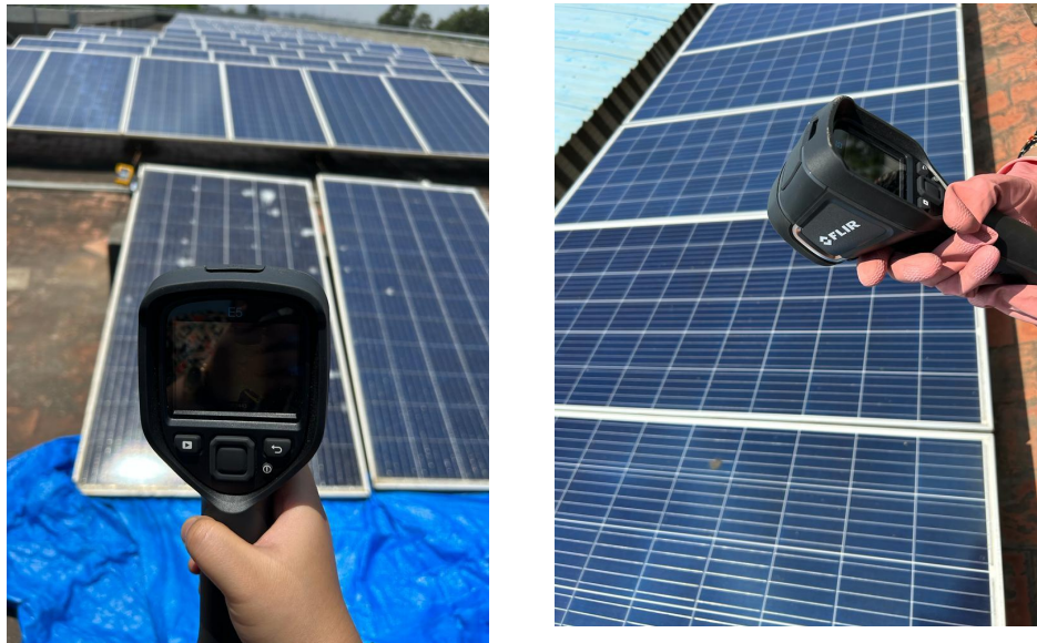
Fig 4.2. On-field usage of FLIR Thermal scanner
